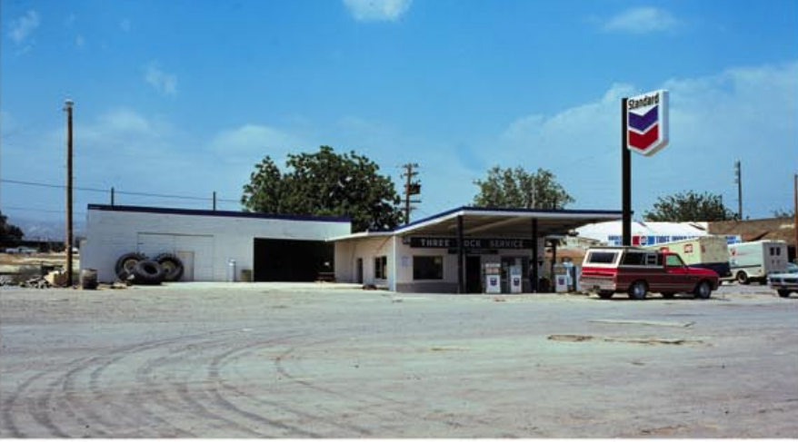
Fig. 14. As water percolated into soil around this gas station at Three Rocks, San Joaquin Valley, California, the station settled into collapsible soil in old earth flow deposits. Notice that as a result of hydrocompaction, the gas station sits below ground level. The pump area did not settle, causing a tilt in the overhanging roof.
