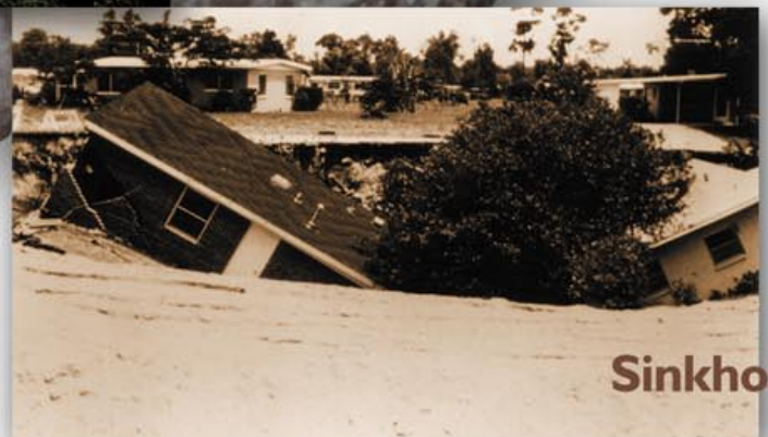
Fig. 3. Catastrophic collapse near Barstow, Florida, in the late 1960's destroyed two houses and formed a sinkhole. Groundwater slowly dissolved the underlying limestone and created an underground cavity into which the ground eventually collapsed.
