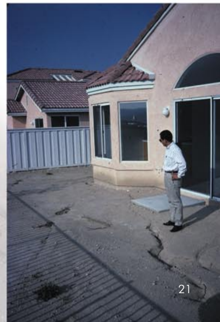
Fig. 15. Cracks caused by hydrocompaction appeared in the Temecula Valley, Riverside County, California, after watering of lawns caused the water table to rise up into collapsible soils.
