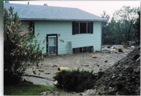
Fig. 25. (Right) A debris flow partially buried and filled this house in Bountiful, Utah, in 1983.
