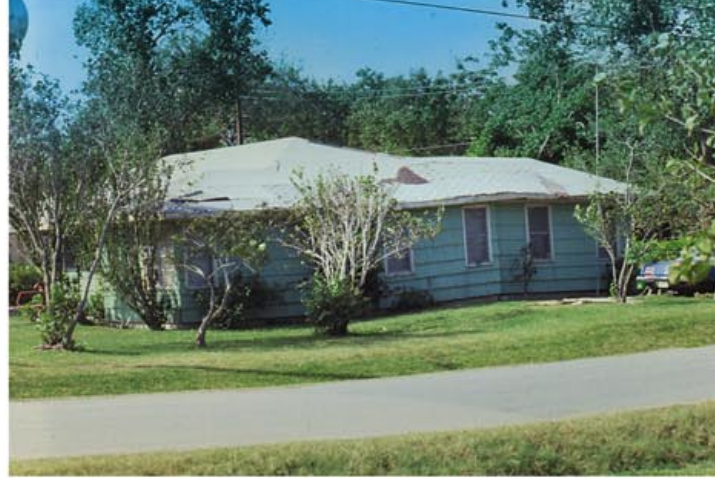
Fig. 39. Surface faulting caused by groundwater pumping damaged and deformed (note eaves) this house in Baytown, Texas, near Houston. The yard was formerly flat and even; the gentle ground flexure is the fault scarp.
