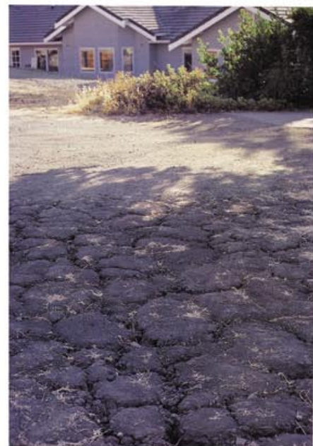
Fig. 11. Expansive soil swells when it is wet and shrinks and cracks as it dries (foreground).
