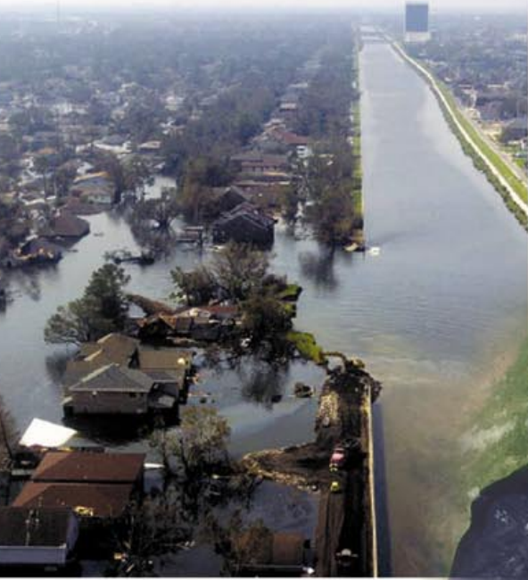
Fig. 10. When the levee failed along the 17th Street Canal in New Orleans during Hurricane Katrina (2005), sliding occurred along a soft clay layer interbedded in organic soil deposits beneath the levee allowing water in the canal to push the levee landward like a giant plow.
