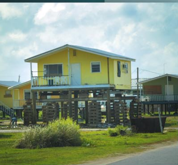
Fig. 48. These homes in coastal Louisiana were elevated to reduce flood damage. Building codes and land-use regulations can require that owners of property build new structures at a specified elevation to avoid flood damage.
