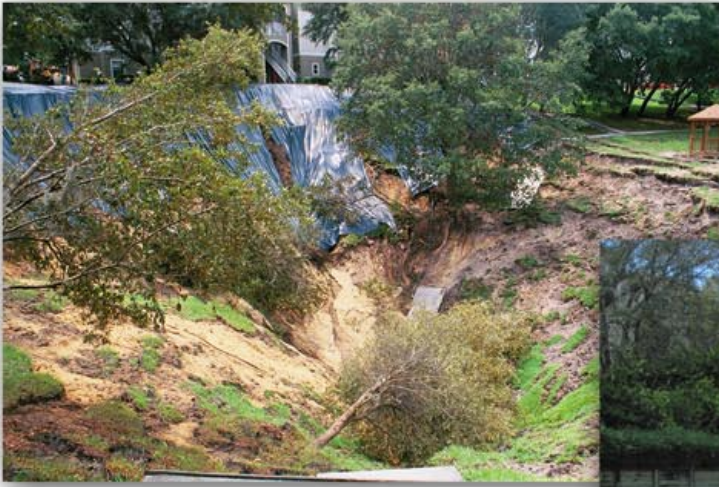
Fig. 31. (Before) Sinkhole that formed on June 11, 2002, in Pine Hills, Central Florida, and created a 150-ft-wide and 60-ft-deep cavity. It forced evacuation of 100 occupants living in apartments in background. (After) Site was permanently stabilized with a 50-ft-deep wall consisting of 3-ft-diameter interlocking piles.
